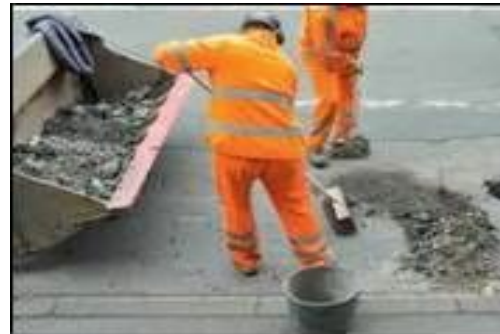
Fill and compact with pothole-fix
