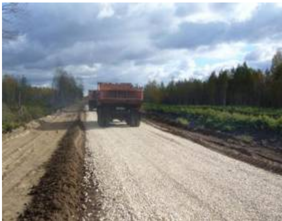
Finished surface with gravel - bitumen layer is missing
