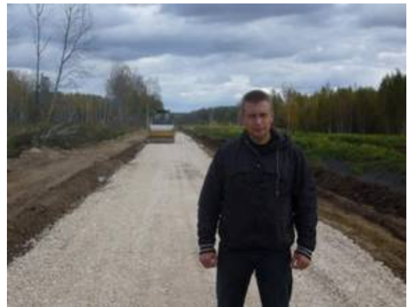
Finished surface with gravel - bitumen layer is missing
