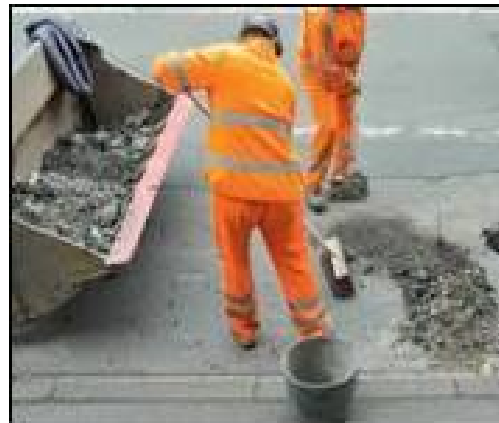
Fill and compact with pothole-fix
