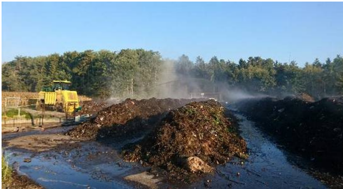
Compost facility in Austria - 8.000m 2 TERRA-3000® -stabilized storage area
