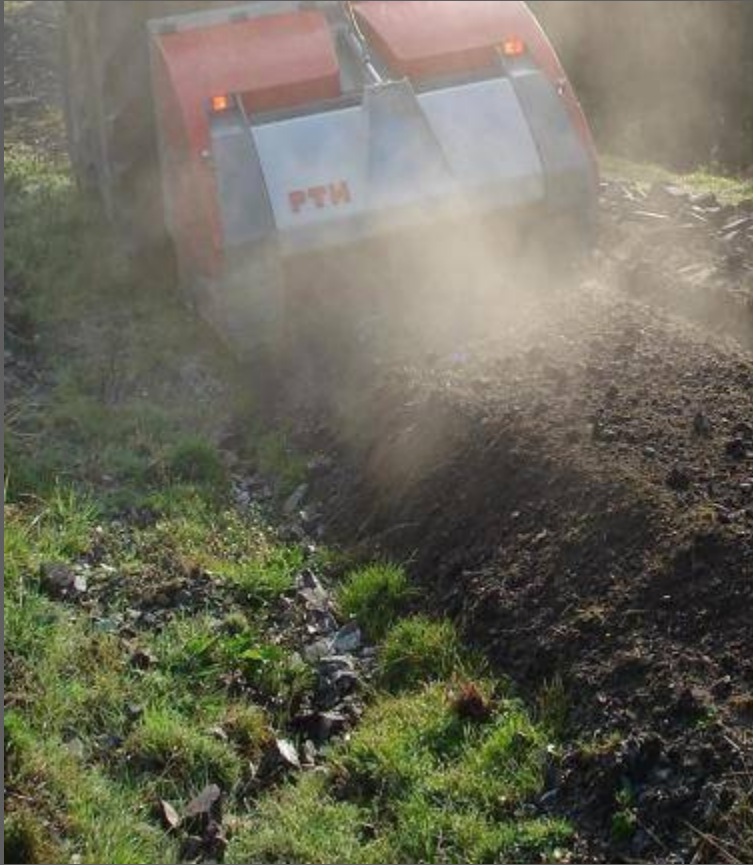
Mixing TERRA-3000® and soil material even by mill or crusher.
