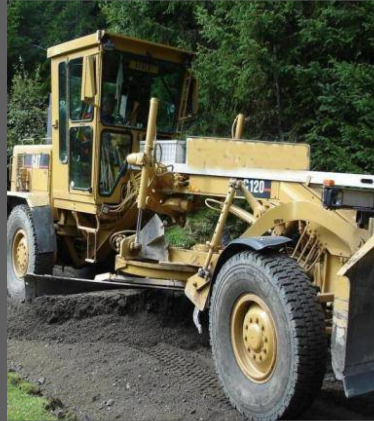
Produce fine level by grader.
