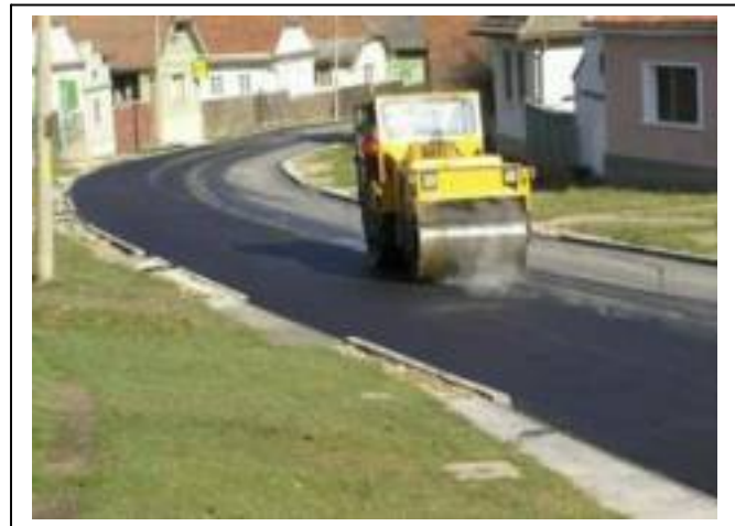
Finally we protect our work with a wearing course.
