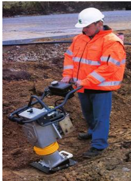
Fill and compact with TERRA-Mixture
